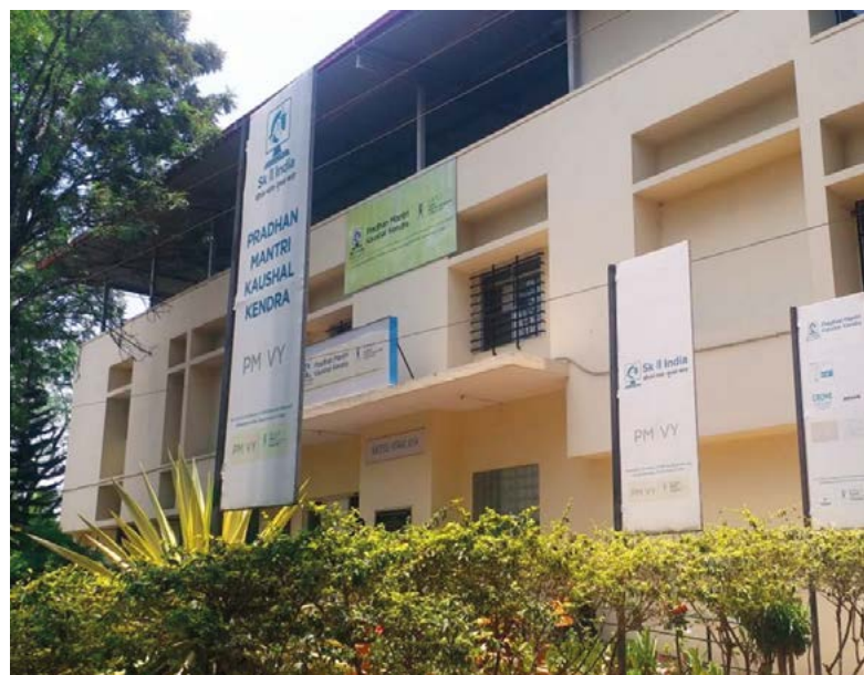
Skill training centre and office for the social work
